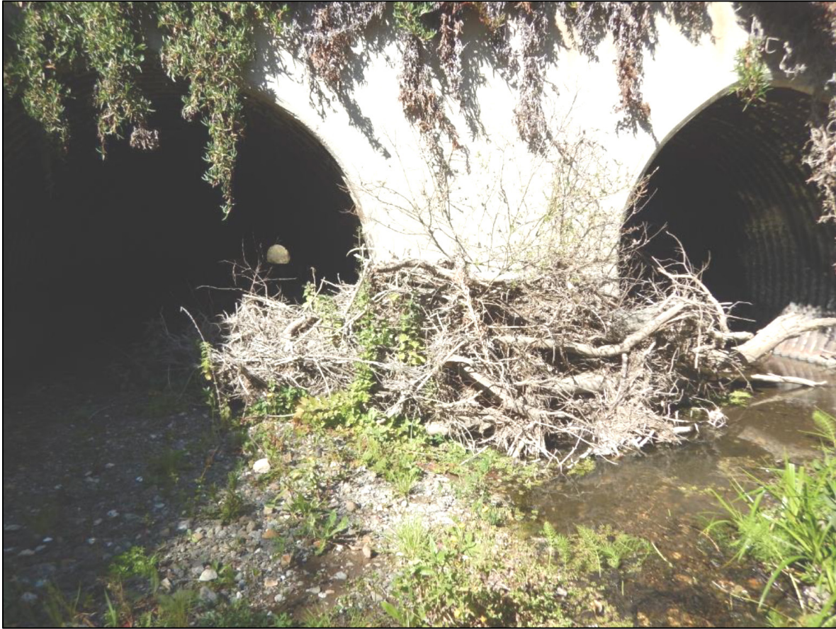
Figure 1-3. Inlet End of the Honda Creek Culverts Showing Trapped Debris and Sediment
