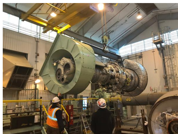
Figure 14 – Delevan Compressor Station Turbine Exchange
