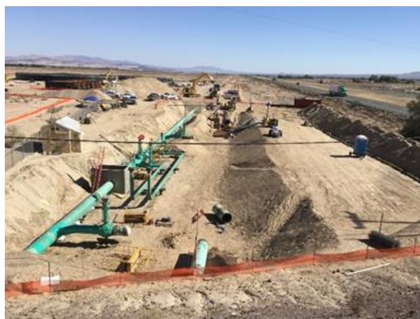
Figure 28 – Strength Test in Progress
