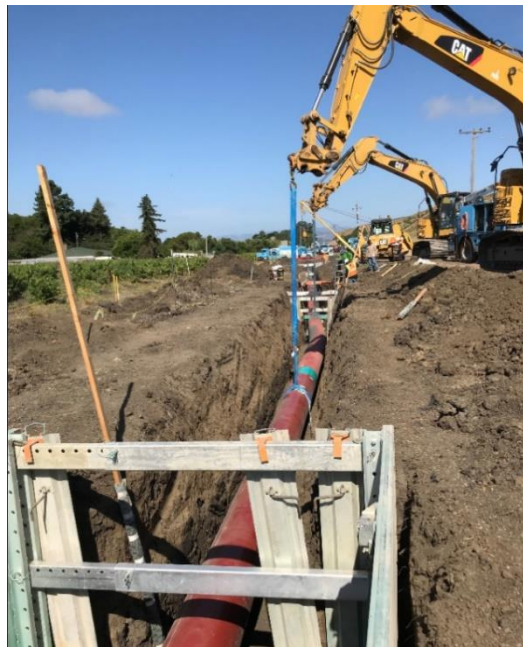
Figure 29 – Vintage Pipe Replaced in American Canyon
