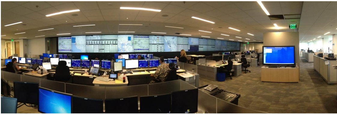
Figure 39 – PG&E’s Gas Control Center Features a 90 Foot-Long Video Wall With Current Operational Information to Augment The Gas SCADA System (Photo Captured Pre COVID-19)
