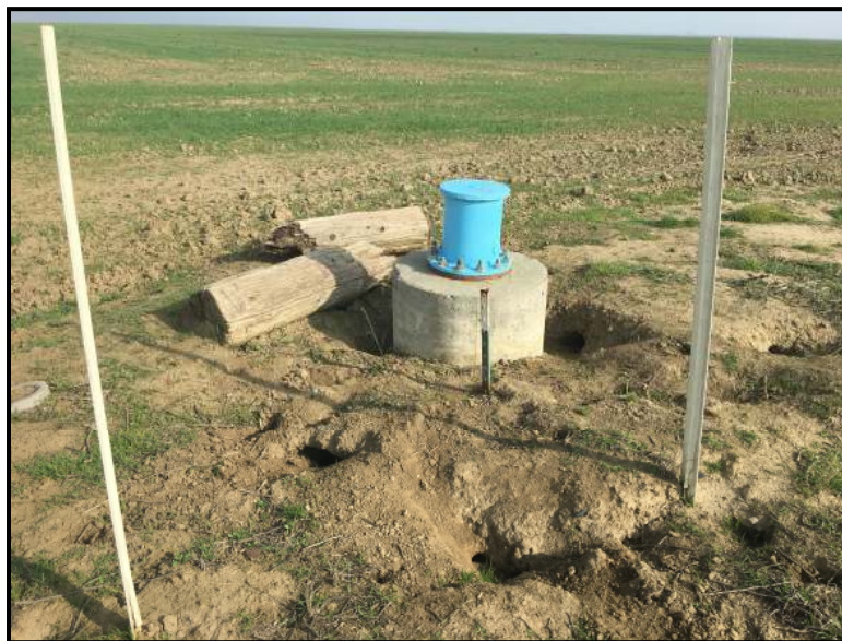
Example of standpipe with steel cap along south boundary of Site
