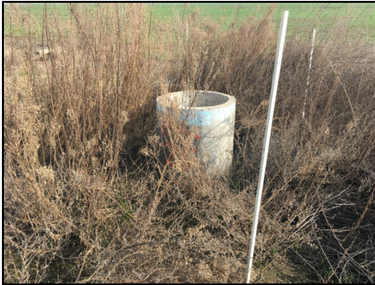
Example of concrete standpipe on Site
