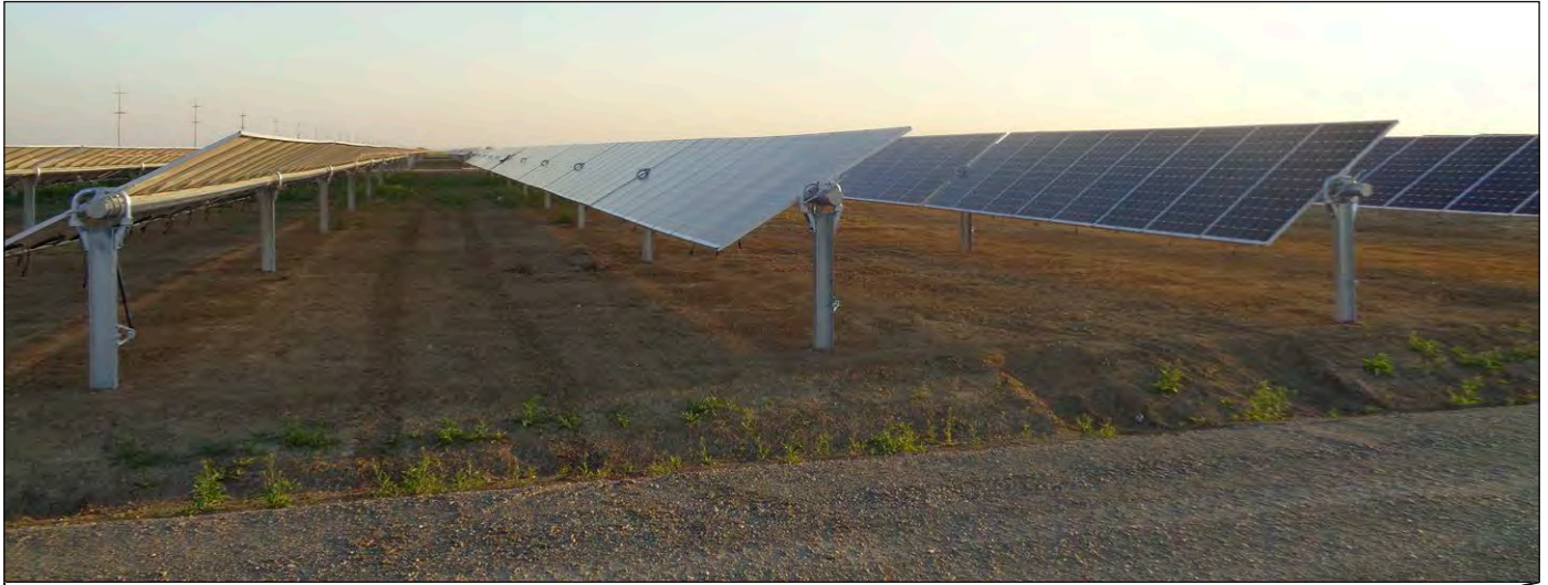
Solar PV Modules on Horizontal Trackers
