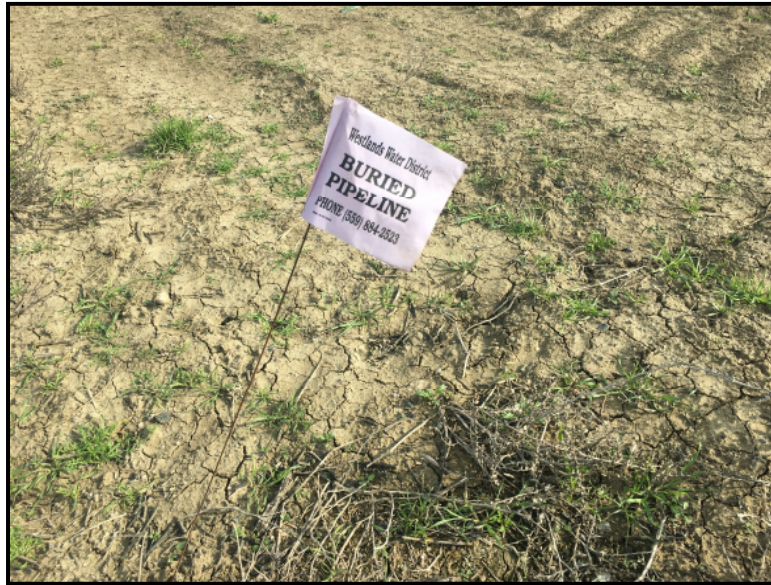
Example of buried pipeline marker on Site
