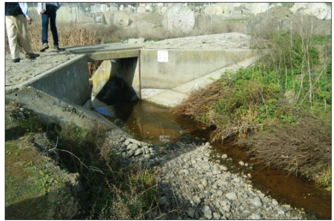
Photo 4. Typical view of an existing drop structure (upstream side) (October 2015)
