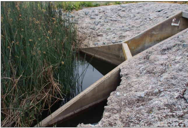
Photo 3. View of drop structure #12 (downstream side) where grouted rock slope protection is proposed to fill void (May 2018)
