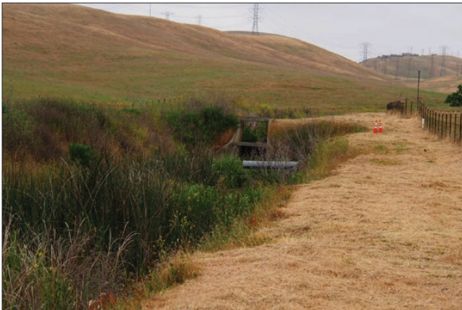
Photo 11. Existing channel conditions near Station 127+00 where significant erosion is evident and full RSP treatment is proposed (May 2018)
