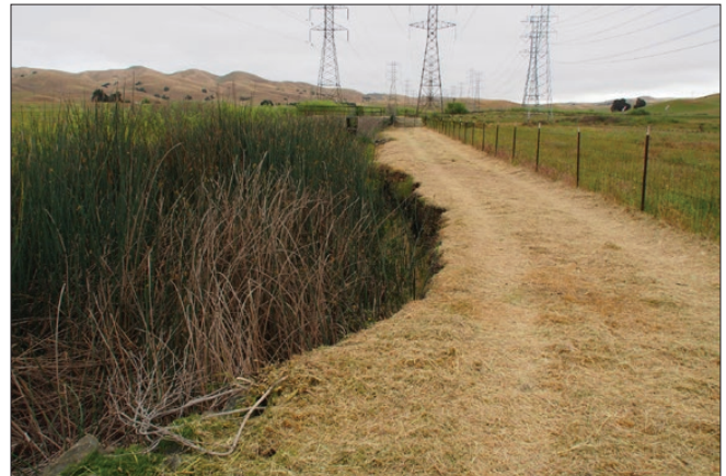
Photo 6. Existing channel conditions near Station 79+00 where substantial bank erosion is evident but roadway width is sufficient. Partial RSP proposed at this location (May 2018)
