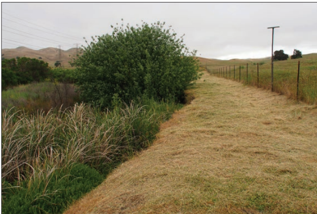
Photo 9. Existing channel conditions near Station 97+00. Treatment methods proposed at this location include vegetation and sediment management as well as willow staking (May 2018)
