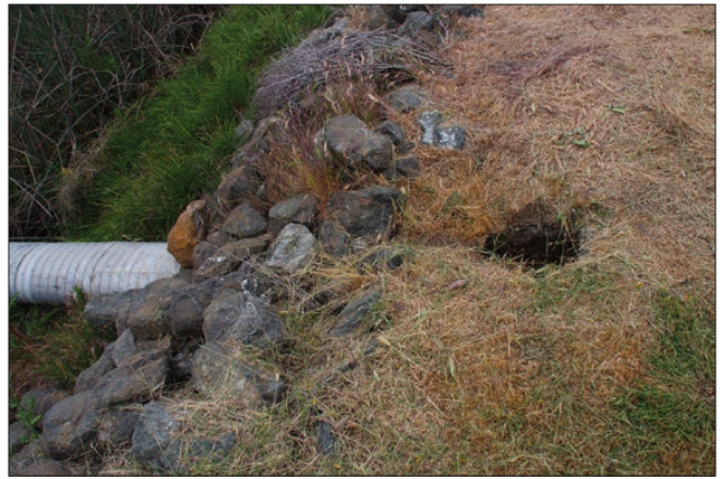
Photo 8. Existing channel conditions near Station 94+00 where rodent burrowing is evident and undermining both the maintenance road and a culvert outfall that drains into Vallecitos channel (May 2018)
