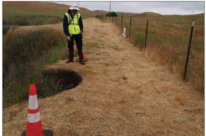
Photo 12. Existing channel conditions between Stations 125+00 and 126+00 where severe bank erosion is evident and the remaining width of the access road is insufficient. Full RSP is proposed at this location (May 2018)
