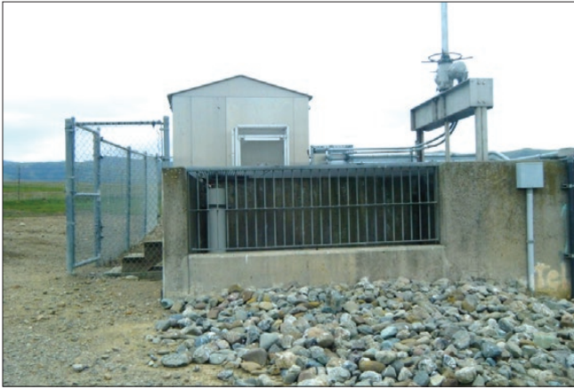
Photo 1. View of channel headworks structure where the SBA pipe transitions to the trapezoidal channel (October 2015)
