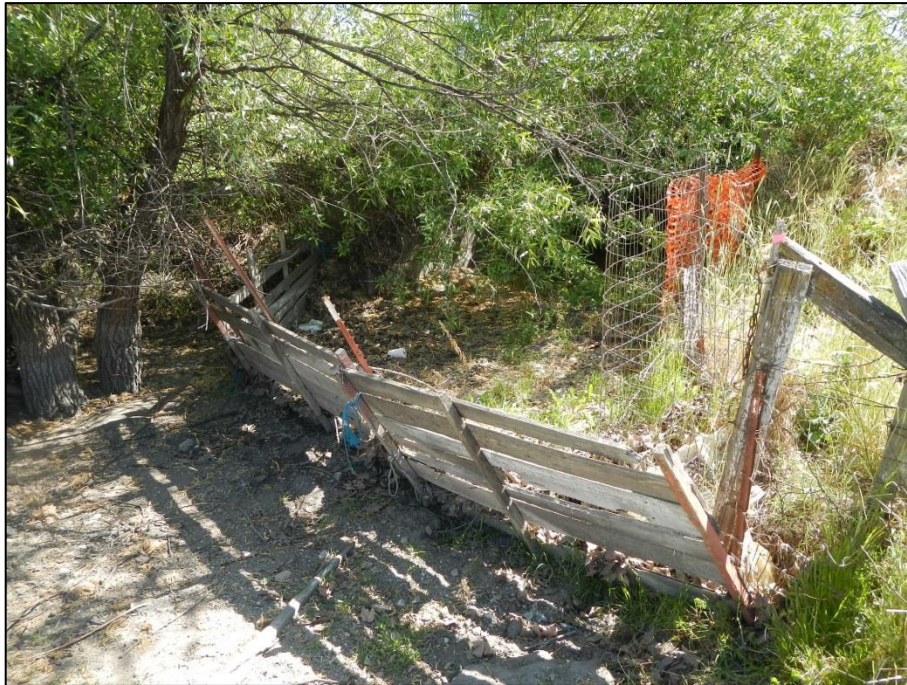
Photo 3. View west of the culvert under Viejo Camino, with a debris rack just downstream of the culvert outlet (May 17, 2018).
