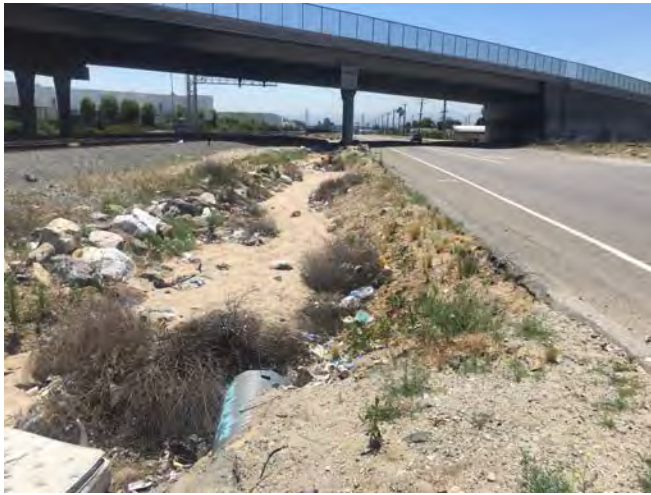
Photo 5. Feature 1 travelling southeast before becoming a concrete-lined ditch for approximately 133 linear feet under University Parkway/North State Street then returning to an earthen-lined channel, continuing off site, and then terminating.
