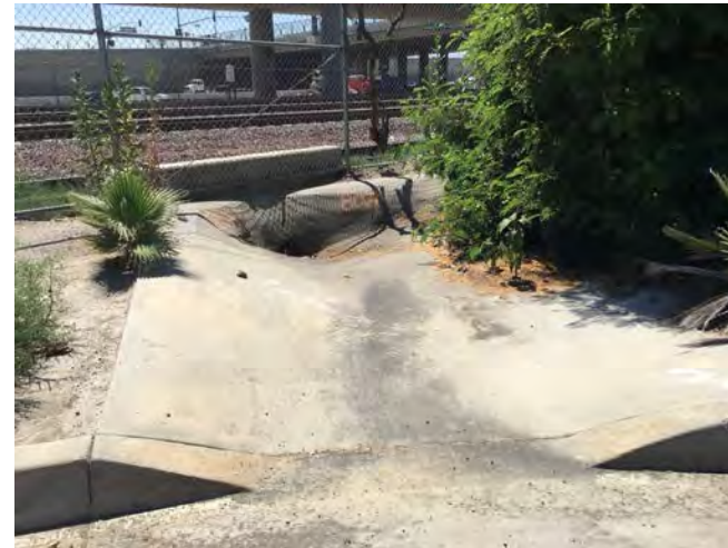
Photo 8. The concrete-lined Feature 2 commences from the road and a culvert under the railroad tracks (shown above) before combining into a single, concrete-lined channel.
