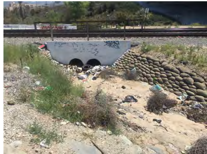
Photo 4. Double culvert on west side of railroad tracks through which Feature 1 travels before continuing southeast along Cajon Boulevard.
