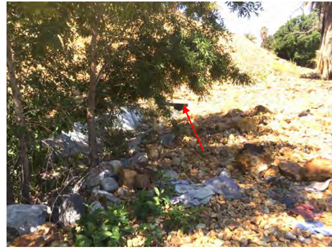
Photo 10. Storm drain inlet (red arrow) where some flows from Feature 2 travel after entering a riprap basin. Other flows continue south before travelling off site and entering another storm drain inlet.
