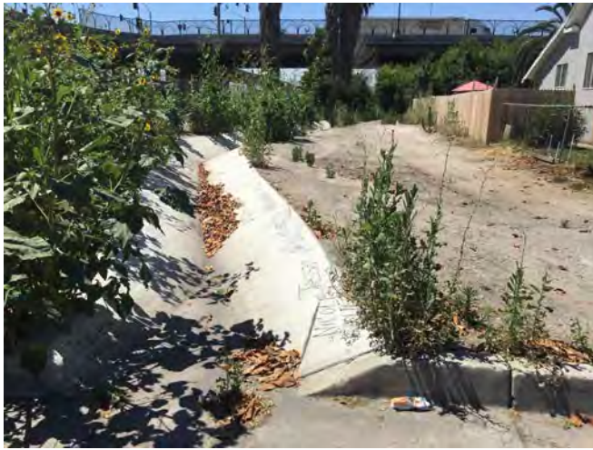
Photo 9. The concrete-lined Feature 2 commences from the road (shown above) and a culvert under the railroad tracks before combining into a single, concrete-lined channel.
