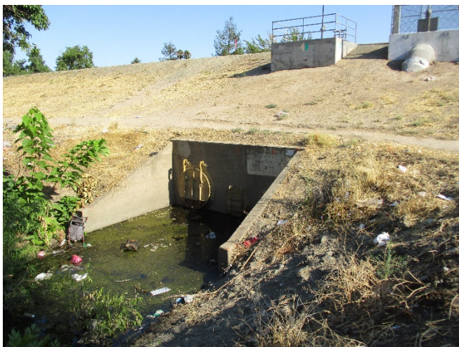
Photo 13. View looking northwest toward the Sump 103 outfall as it enters Arcade Creek. The banks around the outfall have been reinforced with concrete. 23 July 2020.
