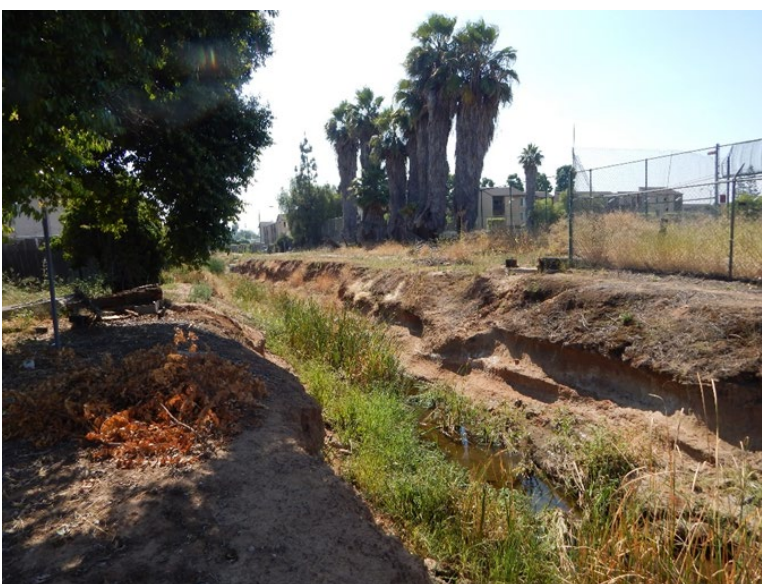
Plate 6. Overview of the bank erosion in the portion of the project alignment east of Ballantyne Street. View to the southeast.
