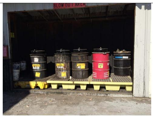
Photo 8: Oil Blow-Out Area containing five 55-gallon drums on secondary containment.
