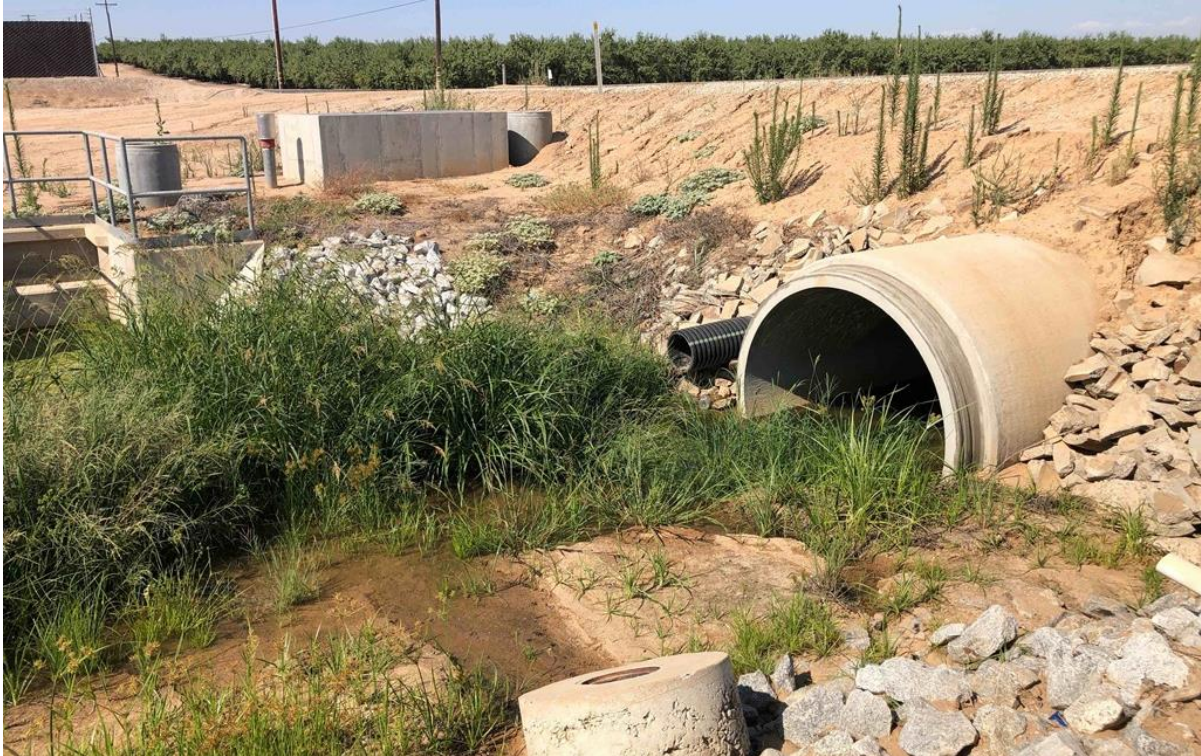
Photo 5. A culvert carries water from Root Creek beneath paved road. (Aspect: northeast)
