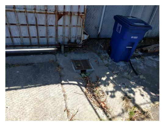
Photo # 4. Storm water inlet. Drains to Tenth Street storm sewer.
