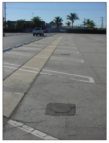
**Photograph 14**: View of concrete strip and patches.
