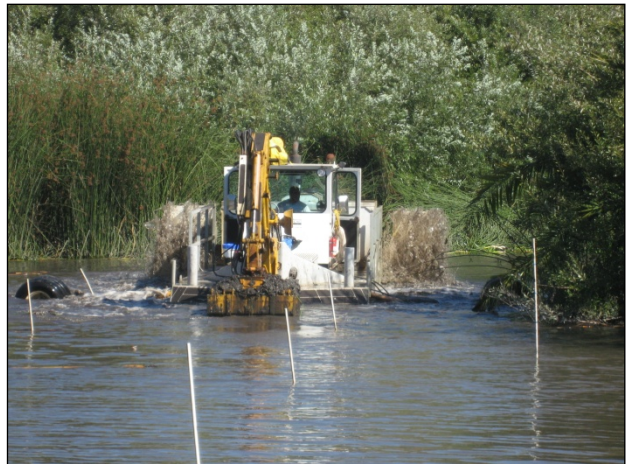
LEFT: Off-loading dredge sediments directly to sealed truck. RIGHT: Channel survey markers define sediment removal area.
