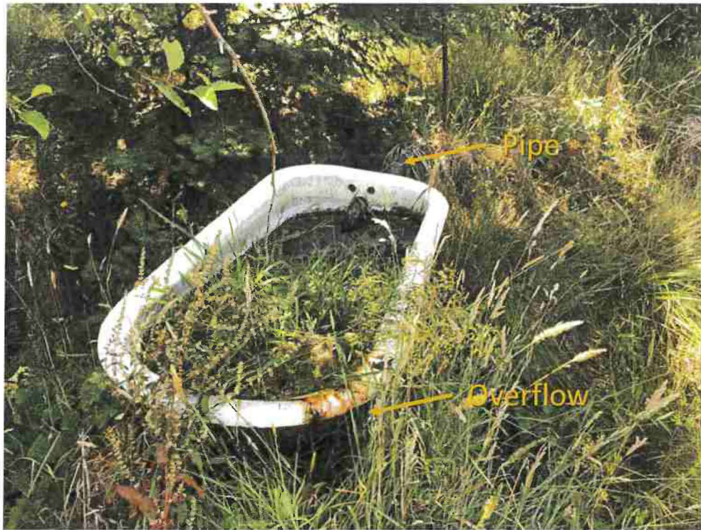
Photo 3. Bathtub cistern filled by shallow well.
