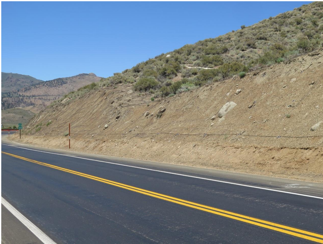
Figure 7 – Color treated Anchored Wire Mesh installed north of project.
