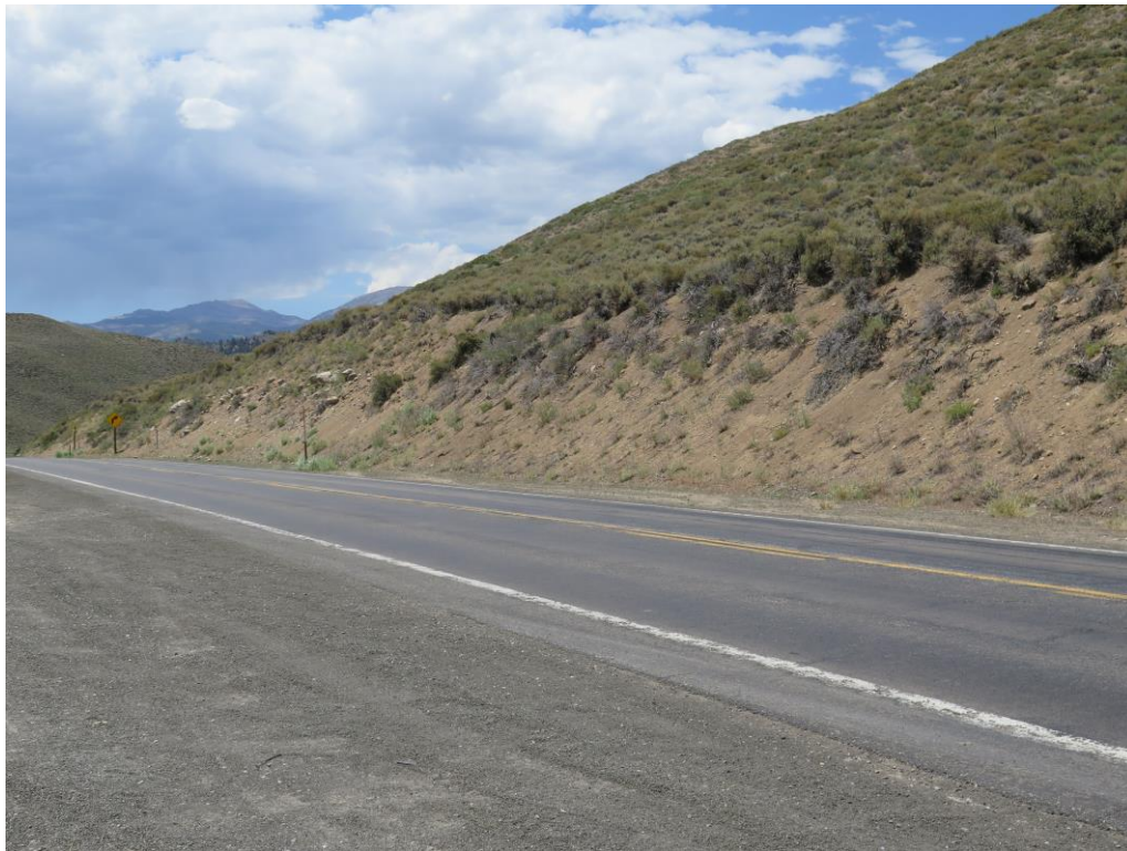
Figure 6 - Existing roadside cut-slope in project limits with minimal to moderate vegetation coverage.
