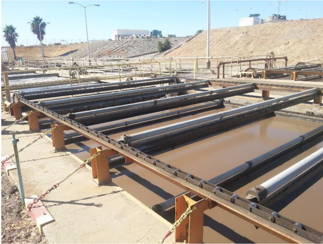
Figure 2-2 Surface Skimmers and Primary Clarifiers
