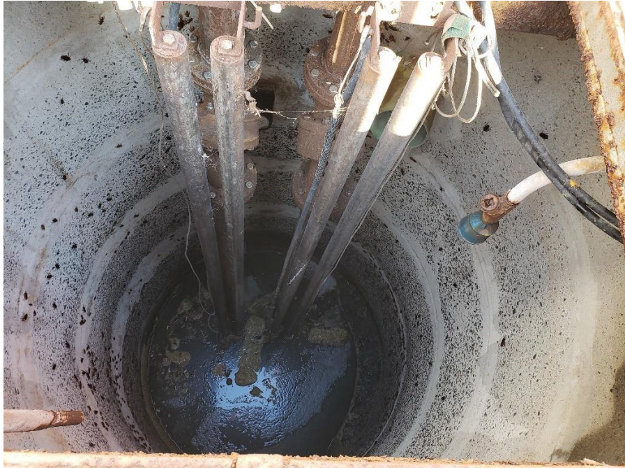
Figure 3-4 Amador Lift Station Wet Well
