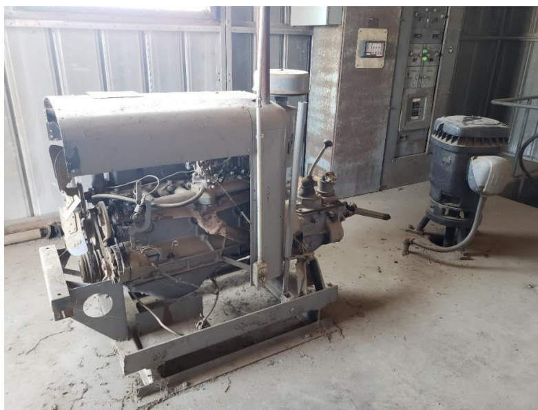
Figure 3-8 Eleventh Street Lift Station Upper Level with Backup Diesel and Vertical Turbine Motor
