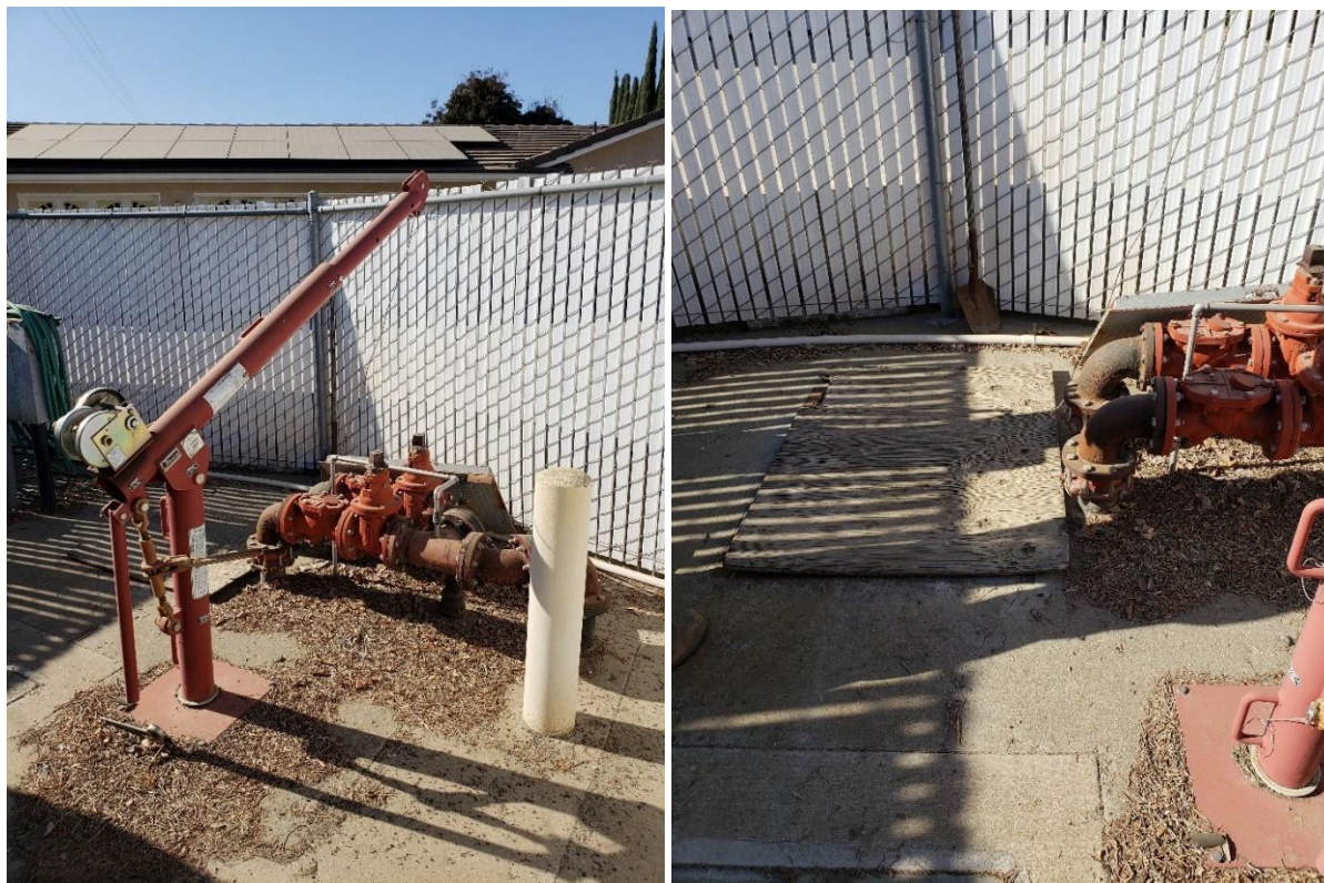
Figures 3-2 and 3-3 Amador Lift Station Pump Hoist with Hand Winch (left), Plywood Pump Chamber Cover (right)
