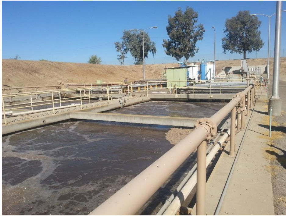
Figure 2-3 Aeration Tanks
