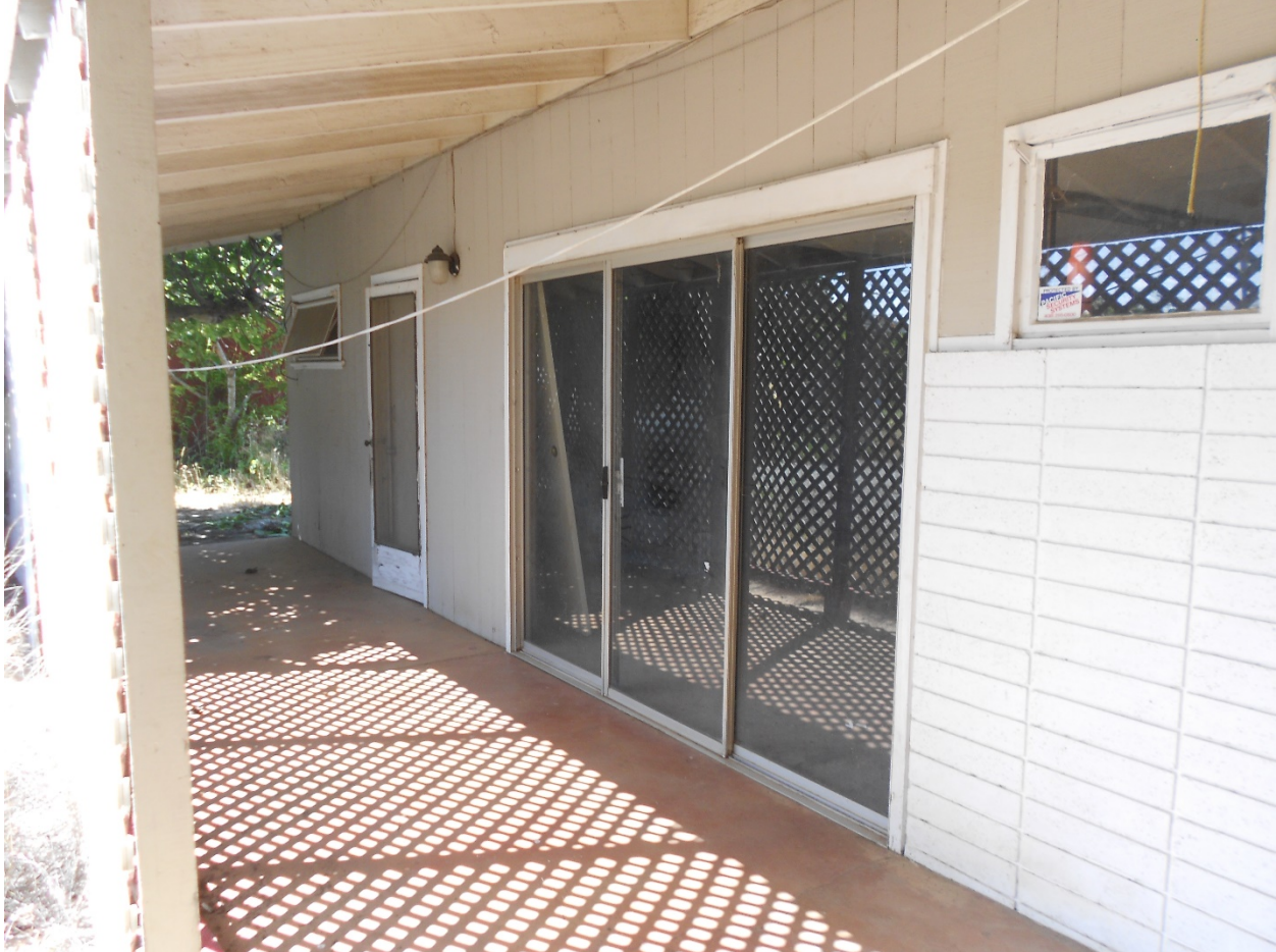
Photograph 2 1105 Half Road, Morgan Hill – Main house View: Front façade, covered concrete porch. Concrete block veneer on the front wall (right). “T-111” Manufactured board siding on the rest of the building.
