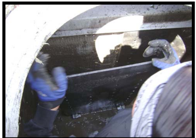
Filter Media Shields Are Removed To Expose BioMediaGREEN Filter Media To Be Cleaned Or Replaced.
