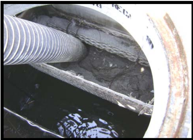
Catch Basin Filters Are Completely Vacuumed Free Of All Pollutants.
