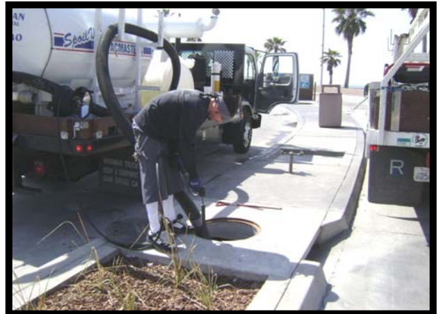
Assess Condition and Pollutant Loading. A Few Gallons Of Water Are Sprayed Into Sediment Chamber To Allow Sediment To Be Vacuumed.
