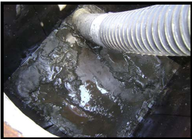
Sediment Chamber Is Vacuumed Clean Of All Accumulated Sediment And Associated Pollutants.
