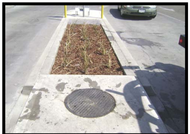
Replace Access Manhole. Check Plants For Growth, Trim If Necessary. Service Is Complete. Total Service Time = 45 Minutes.
