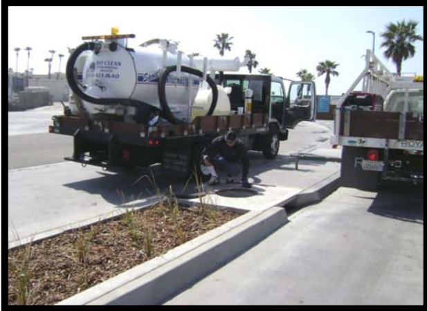
Service Crews Arrive On Site And Remove Access Manhole To Perform Maintenance Service.
