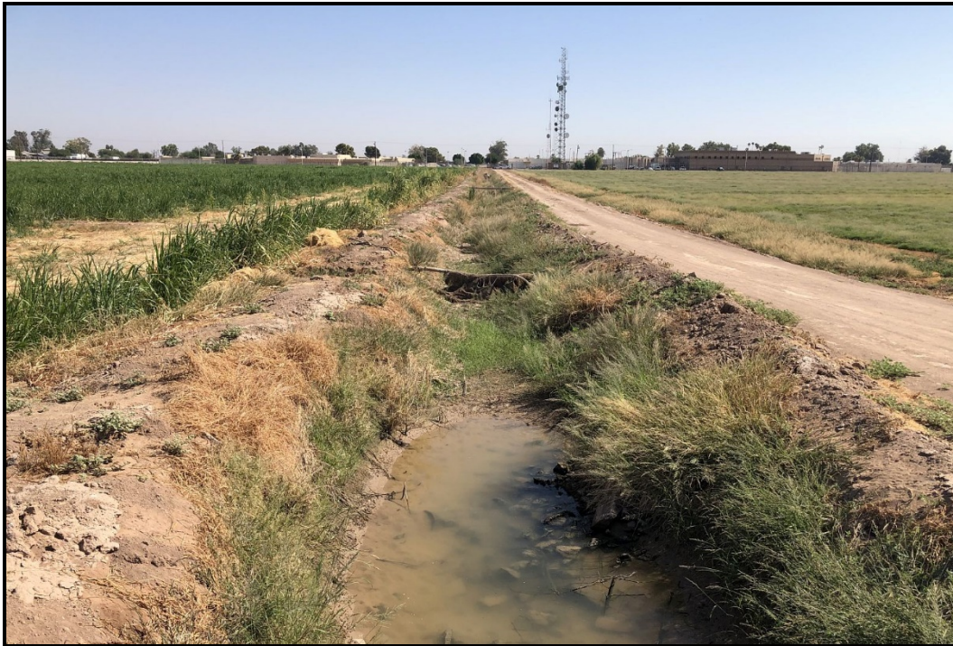
PHOTOGRAPH 5 The Northern and Earthen-Lined Interior Canal that Bisects the Project Area, Looking East
