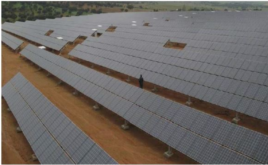
Typical Fixed-Tilt Solar Panel Rows
