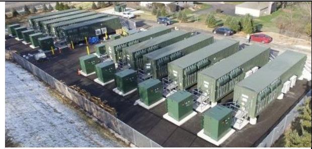
Modular ESS Installed on Concrete Pad
