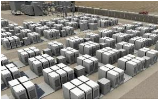
Modular ESS Installed on Multiple Concrete Pads
