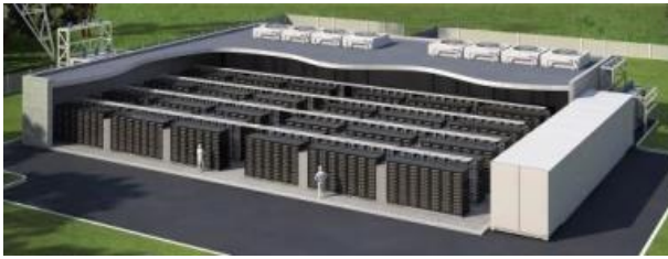
ESS Installed in Dedicated Structure
