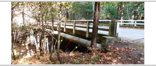
**Exhibit 11.** View of the NCP (red arrow) showing the existing hangars (yellow arrows) supporting the pipeline as it crosses beneath the Newell Creek Access Road Bridge, view looking northeast (DSCN6306)
