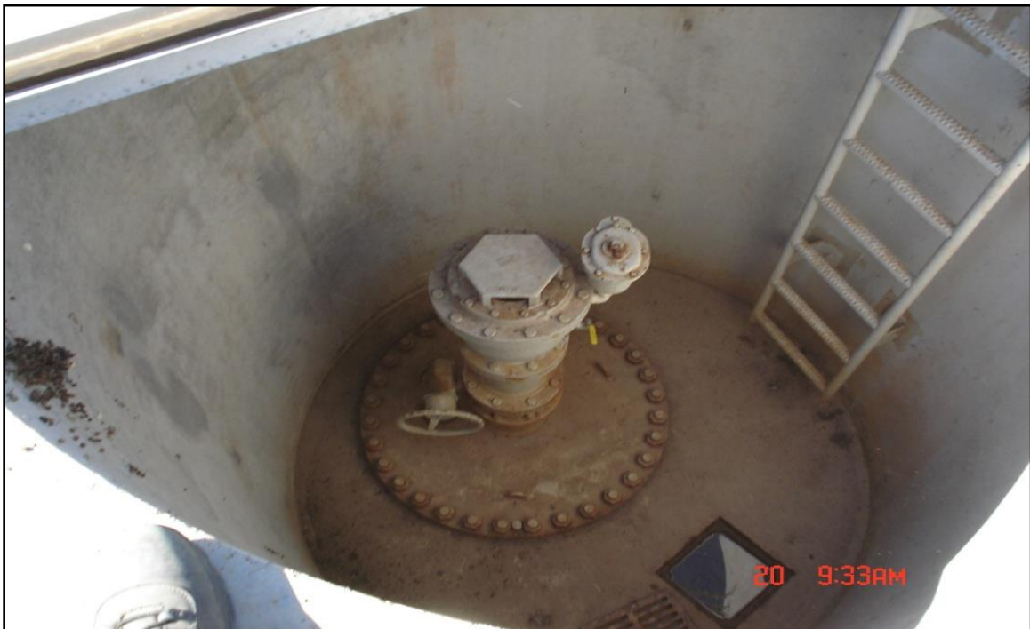
Vault with Air Release Valve
