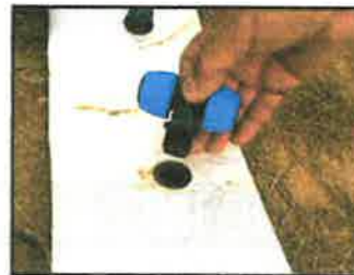
TEE START CONNECTOR THREADS INTO INTEGRAL WELDED OUTLET
