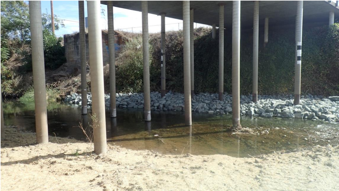
Figure 5A. Due to erosion issues at the bridge, some emergency repairs have already completed directly beneath the bridge and fresh rip-rap has been placed.
