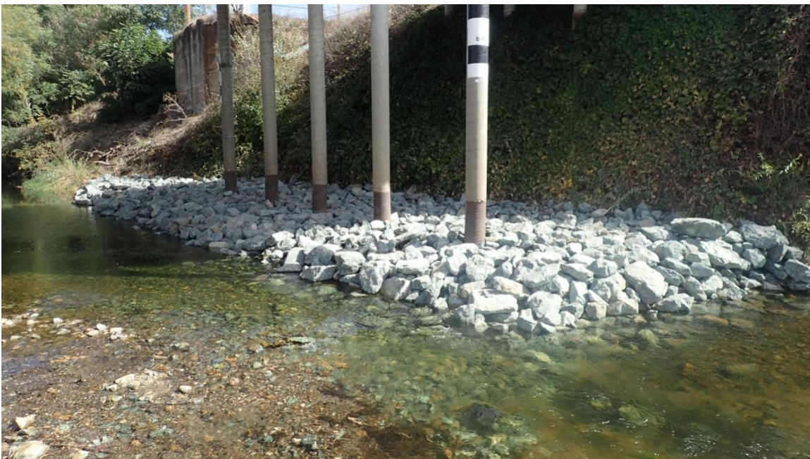
Figure 6A. Close up of the instream component of the emergency repair. Rip-rap intrudes into the thalweg, reducing wetted width at base flows.
