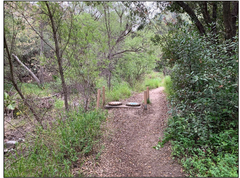
b. Clean-out no. 3 to be replaced with manhole (Station 13+48)
