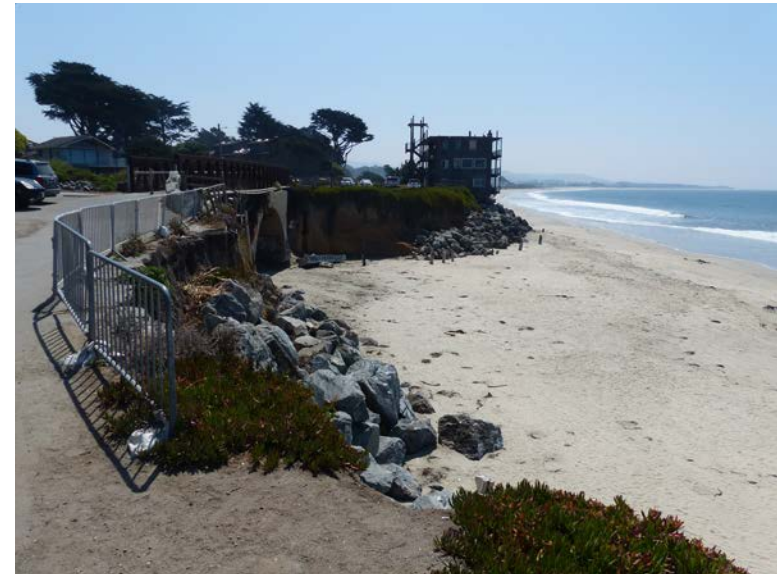
Photo 8. Existing Rock Slope Protection.
