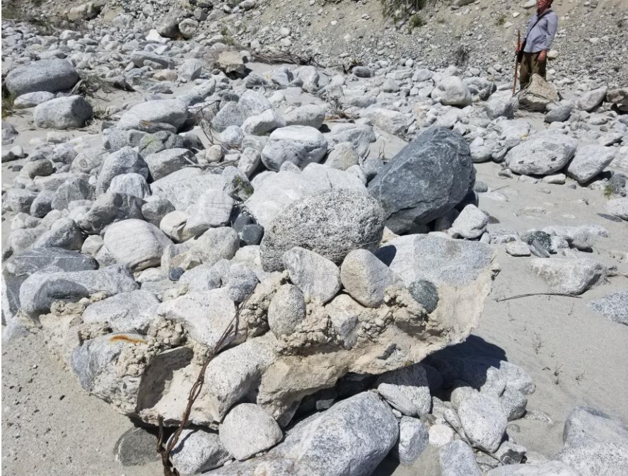
Photo 3: Concrete Matrix Washed out of Whitewater Levee (View E)
