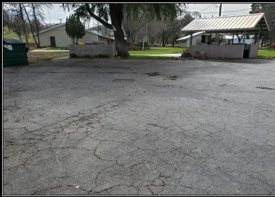
Figure 9: Failing Asphalt That Will Be Replaced (Just South of New Kitchen)
