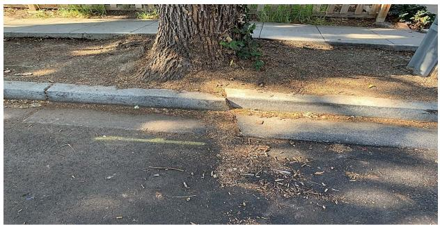
Image #10 – Tree T96, camphor. Note curb and gutter separation due to root diameter expansion.
