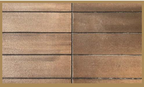
Concrete deck with tight sawcut pattern
