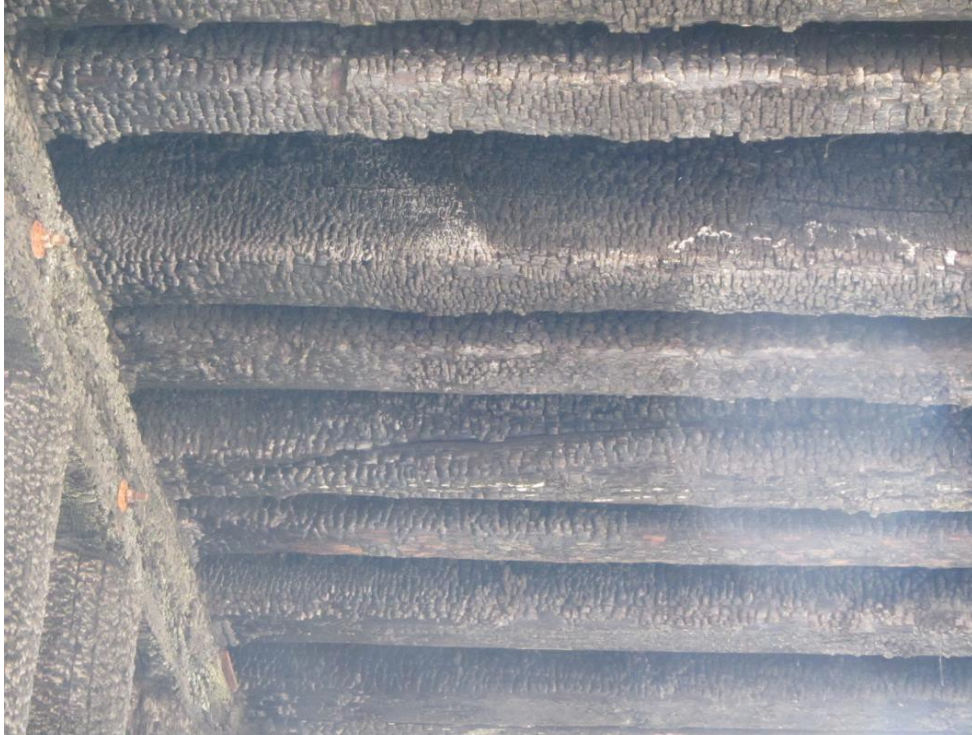
Photo 2: Typical stringer span fire damage.
