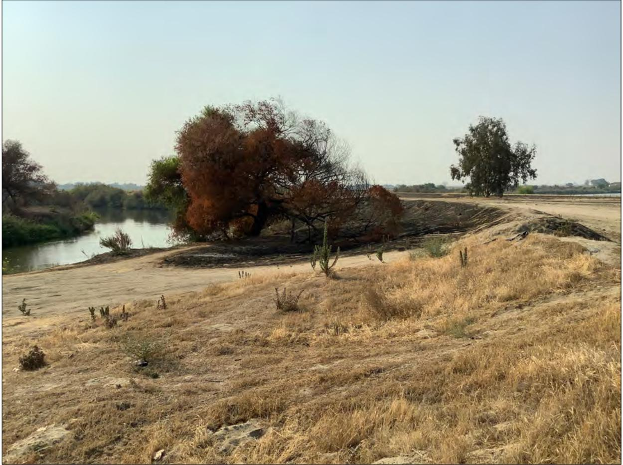
**Figure 6.** Photograph of a berm and the high terrace of the San Joaquin River near Lake Joallan (visible at far right), looking south, showing breaches in the berm that do not provide adequate flood protection for the City.
