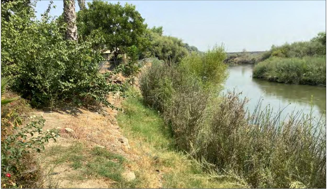
**Figure 9.** Photograph of the Project site, looking north, downriver, showing an eroded riverbank along the San Joaquin River in front of a hotel in Area 2.
