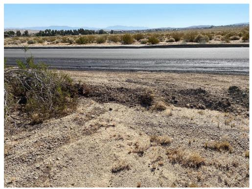
**Photo 8**. Looking northeast (downstream) at Drainage 3. Photo shows that this drainage does not currently leave the site and is blocked by a berm on the west side of Adobe Road.
