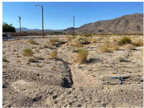
Photo 1. View of Drainage 1 looking south (upstream). Note that the OHWM does not continue past the berm along the south side of Sullivan Road.
