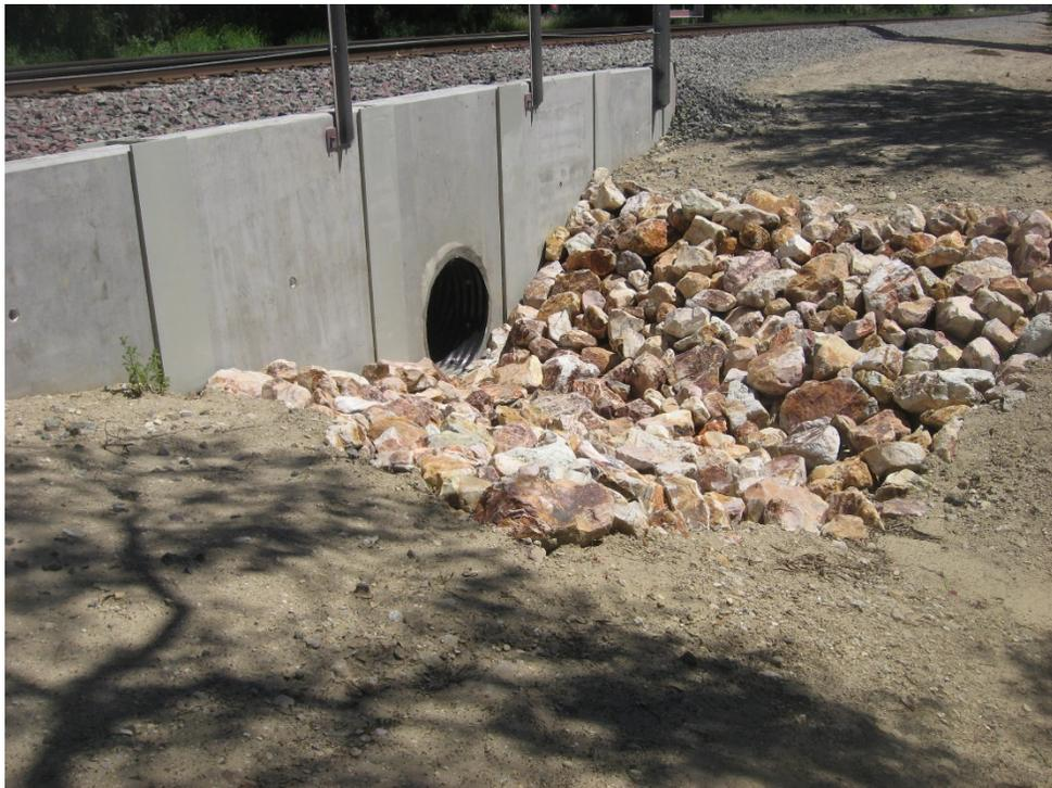
Photograph 14: Outlet of existing culvert MP 436.96 passing beneath the rail looking northeast. No OHWM, bed or bank present (4/21/2020).
