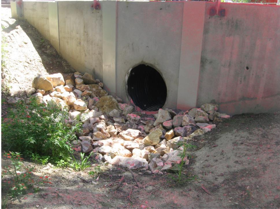
Photograph 13: Inlet of existing culvert MP 436.96 passing beneath the rail looking south. No OHWM, bed or bank present. Based on historic topographic maps, this location did not support a defined drainage (4/21/2020).
