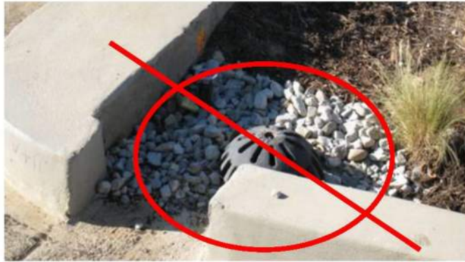
Figure 5: Incorrect Placement of an Overflow Inlet
