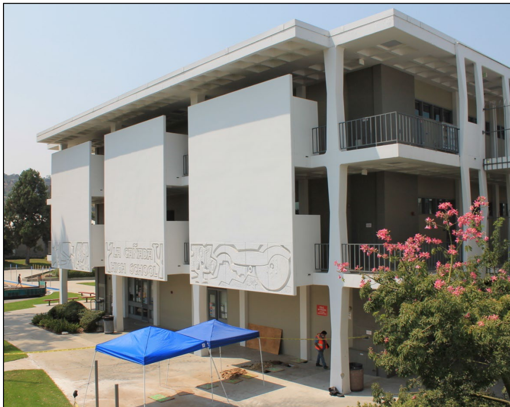
Figure 5: East elevation of Building A with cast-concrete panels. View looking southwest.
