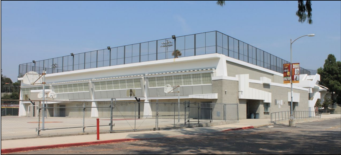
Figure 22: South and east elevations of South Gym. The southern end of the east elevation and the south end of the gym were altered when the open-air, covered basketball court was enclosed.
