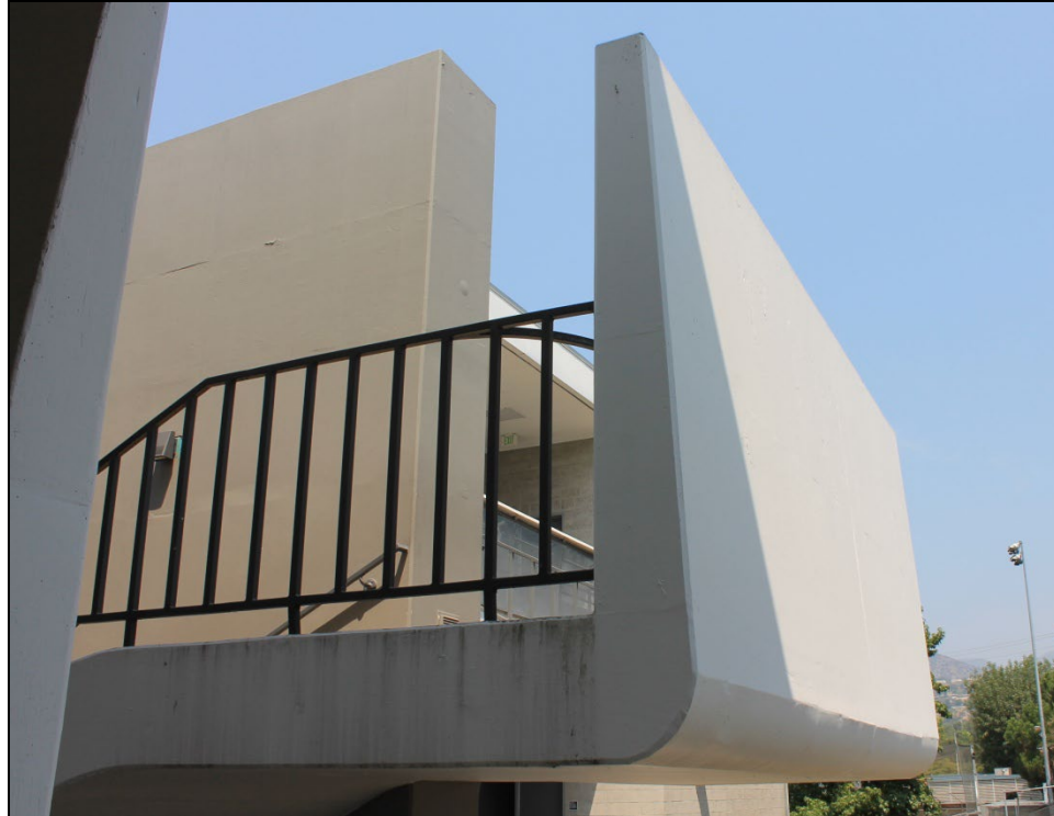
Figure 6: Detail of cast-concrete stairwell located between Buildings A and B.
