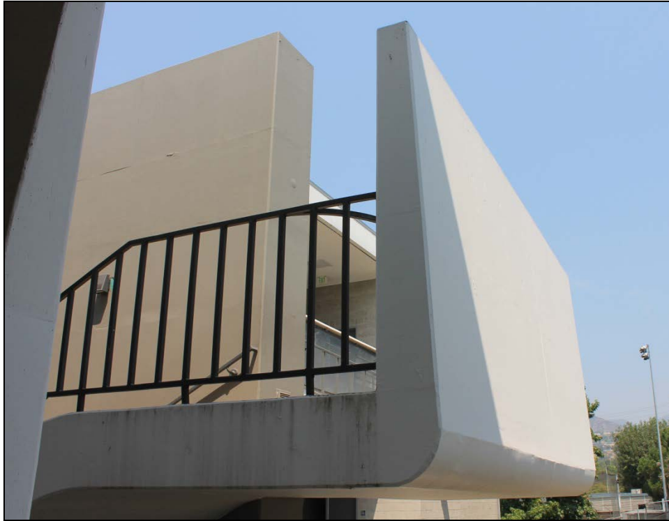
Detail of cast-concrete stairwell located between Buildings A and B.
