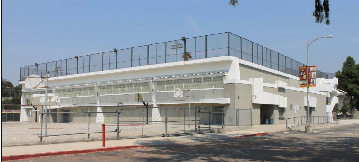
South and east elevations of South Gym. The southern end of the east elevation and the south end of the gym were altered when the open-air, covered basketball court was enclosed.
