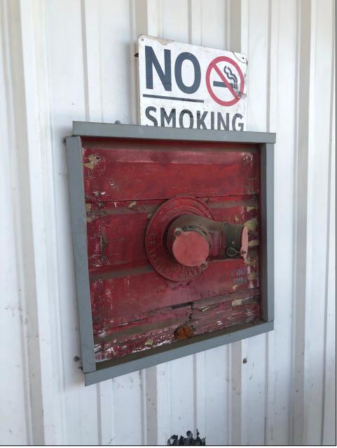
Detail of the original redwood shiplap siding and water hose connection.
