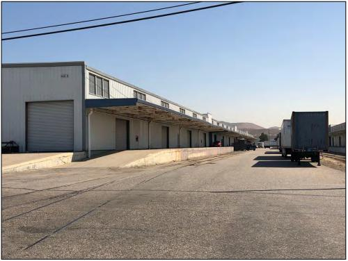
View east of the south elevation showing concrete loading dock and metal doors.
