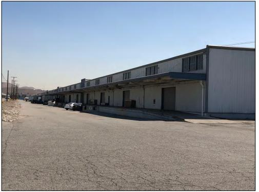
View southeast of the north elevation concrete loading platform and redwood awning clad in metal.
