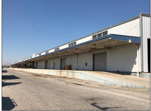
View northwest of the south elevation showing the concrete loading platform and redwood awnings clad in metal.
