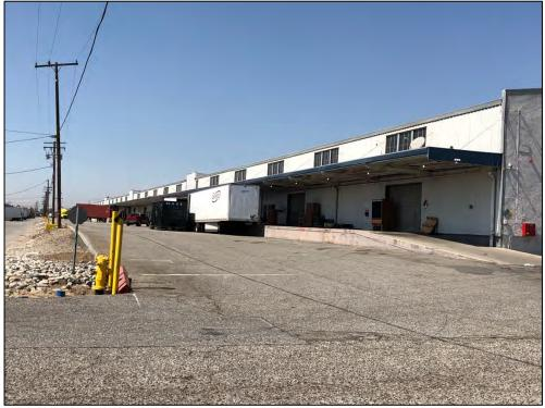
View northeast of the south elevation showing the concrete loading platforms, large openings and awning overhangs.
