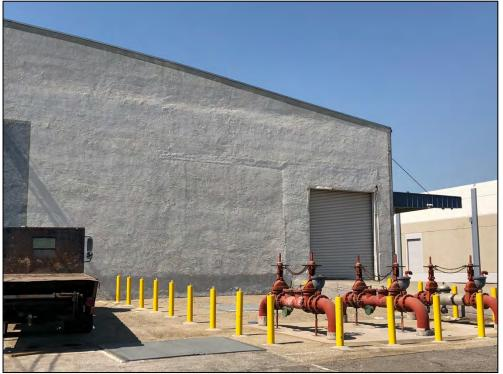
View west of east elevation showing visible indentations in stucco from former openings.
