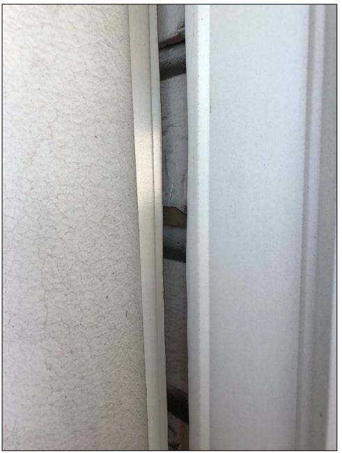
Detail of the original redwood shiplap siding underneath the corrugated metal sheets.
