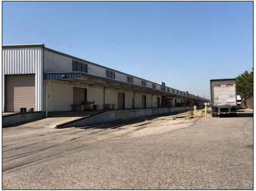
View southwest of the north elevation concrete loading platform and redwood awning clad in metal.
