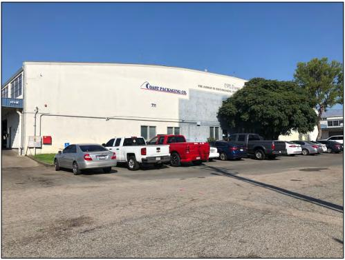
View northwest of the east elevation showing the stucco siding and fixed pane windows.
