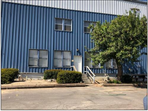
Detail of east elevation entrance and aluminum sash windows.
