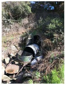
Figure 2 - Collapsed Pipe Sections
