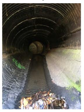
Figure 3 - Inside View of 60-inch CMP Pipe
