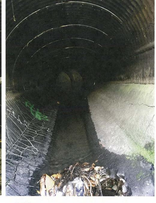
Photo 1: Segments of 60-inch CMP which were undermined by erosion and collapsed into the erosion scar area; corrosion was noted on the inverts of the collapsed segments of CMP.
