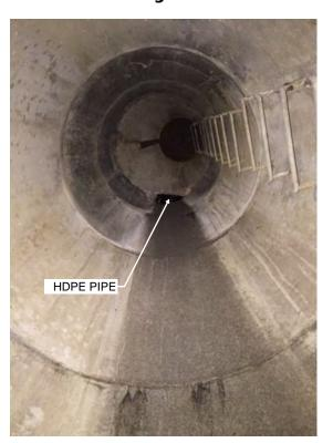
Figure 4 - Inside View and Surface View of Manhole
