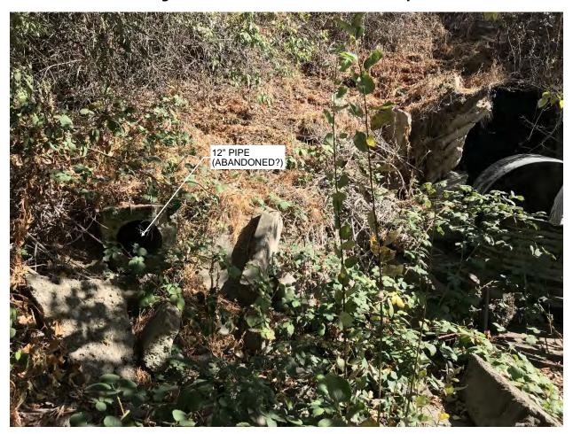
Figure 6 – 12-inch Concrete Encased Pipe
