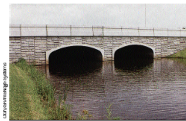
Figure 2. Small bridges may lack the drama of major structures, but they can make an important aesthetic statement when carefully detailed. The precast arch boxes of this bridge in Jacksonville, Fla., have a span of 24 feet and a rise of 10 feet. The crisp line of the arch is complemented by the ashlar stone pattern of precast headwall sections that are tied back into earth fill over the arches. Precast safety railings supported atop the headwall are proportioned to further enhance the overall effect.
