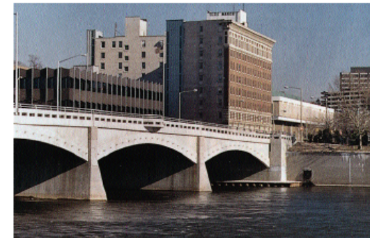
Figure 3. Standard precast, prestressed I-beams support the Bridge Street Bridge in Grand Rapids, Mich. By incorporating precast arch-shaped fascia panels, they maintain a semblance of the old arch bridge that was replaced and harmonize with other bridges in the downtown area.
