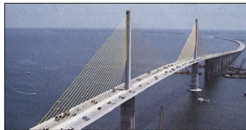
Figure 4. Will the Sunshine Skyway Bridge become a signature structure for the Tampa Bay area, as predicted by the St. Petersburg Times ? This cable-stayed concrete box girder bridge is a prime example of the newest technology for long-span bridges, offering economy of construction that frequently supplants older bridge types. The great variety of possible cable and pylon tower configurations offers designers broad scope for imaginative aesthetic solutions.
