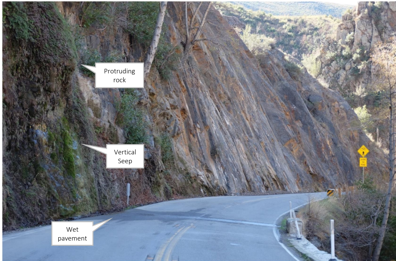
Figure 8. Wet Pavement caused by Springwater and Protruding Rock on Roadway
