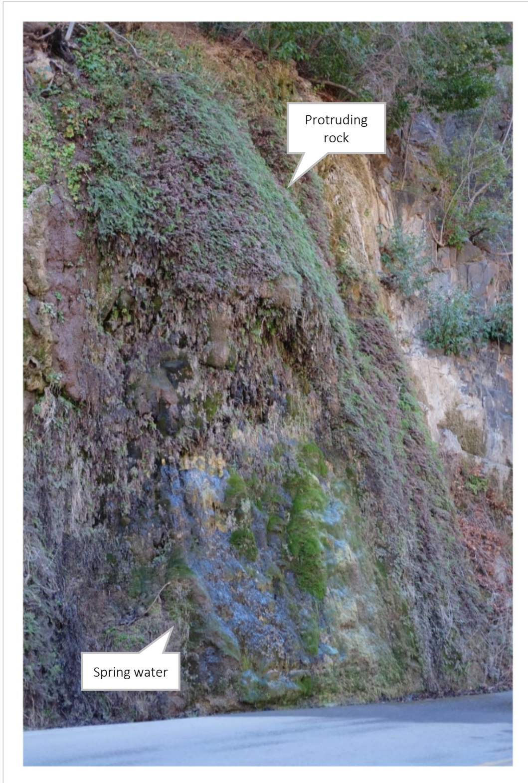
Figure 9. Protruding Rock and Springwater
