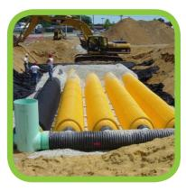
StormTech Isolator Row with Overflow Spillway (not to scale)
