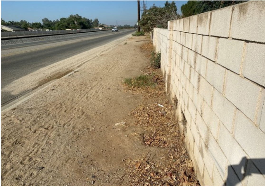
Photo 5. Facing east down Jurupa Rd at the terminus of the Pyrite Channel. Showing cinder block wall that stops flows of the Pyrite Channel.
