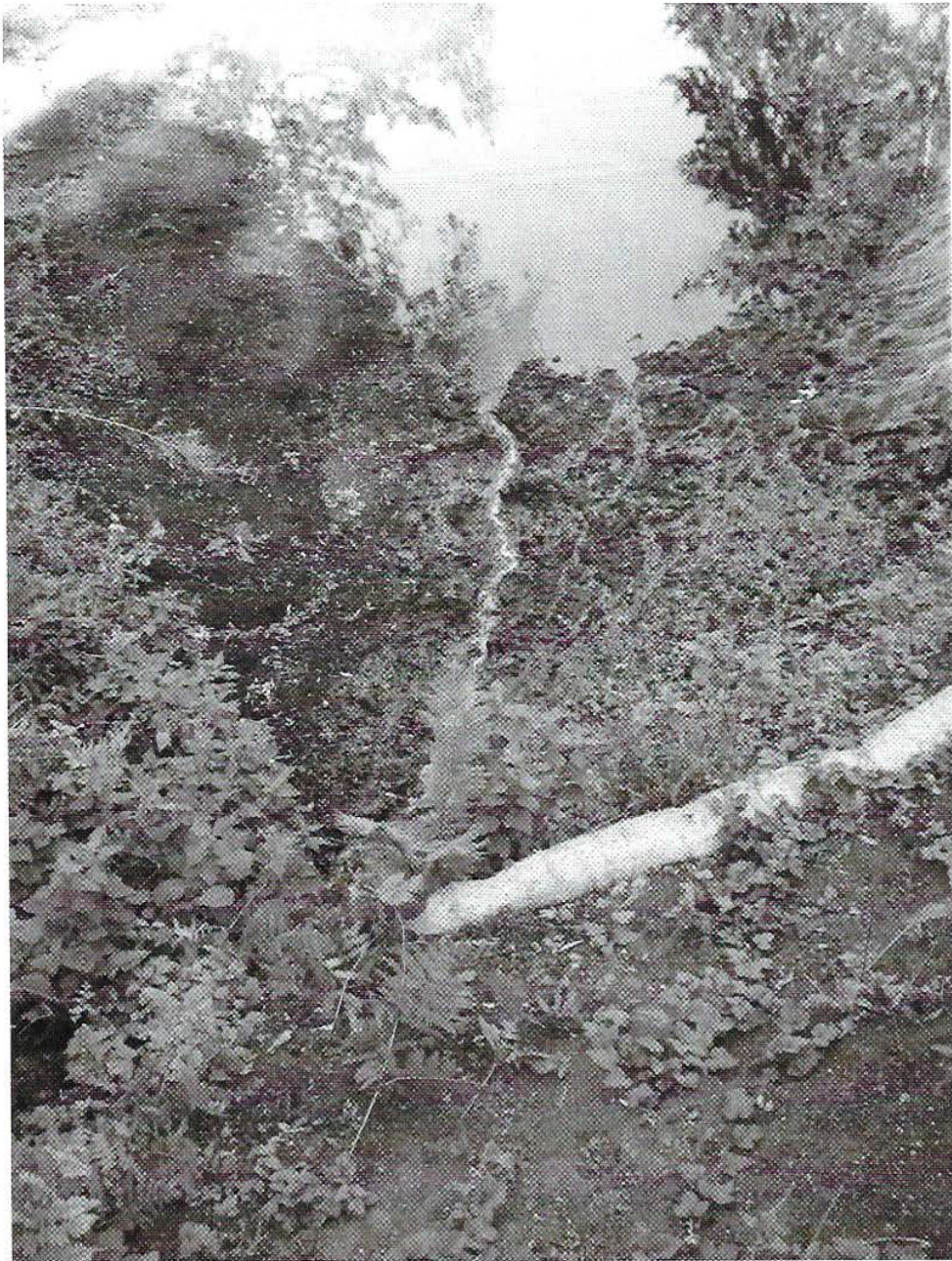
Photo 6. A culvert conveys from a spring to the pond.
