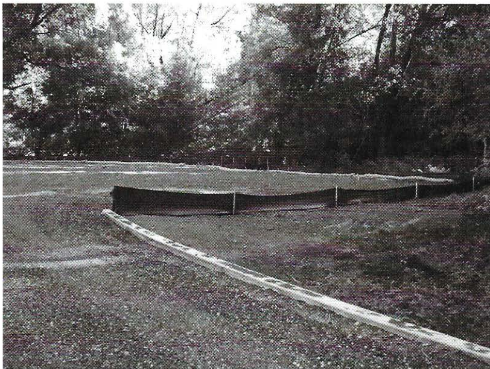
Photo 4. Dirt and gravel pad, presumable made from excavated fill when the pond was created.
