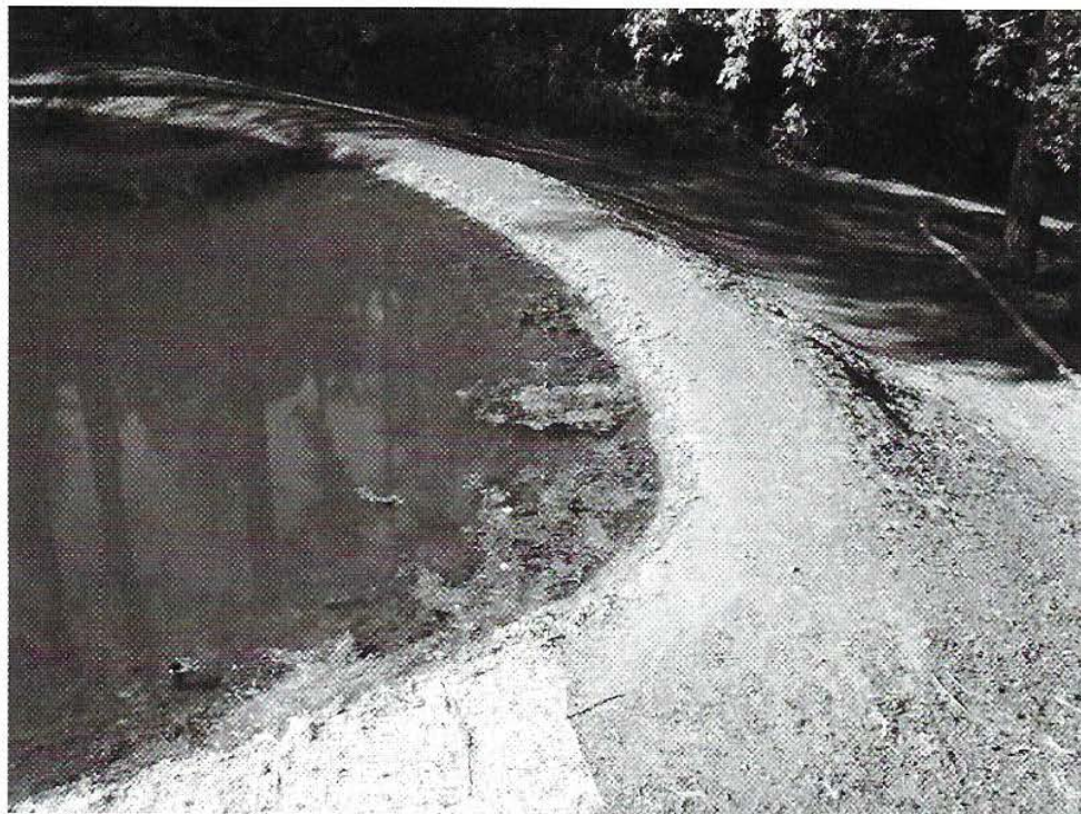
Photo 8. The pond's earthen berm. One of the vertical pipes for outflow can be seen in the bottom left.
