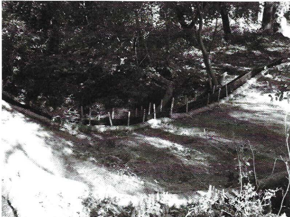
Photo 9. The toe of the berm, erosion control netting and seeding that has sprouted. The culvert discharges into drainage B just below the silt fence.
