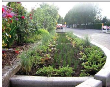
Street-end biofiltration with planting/storage media Source: City of Portland
