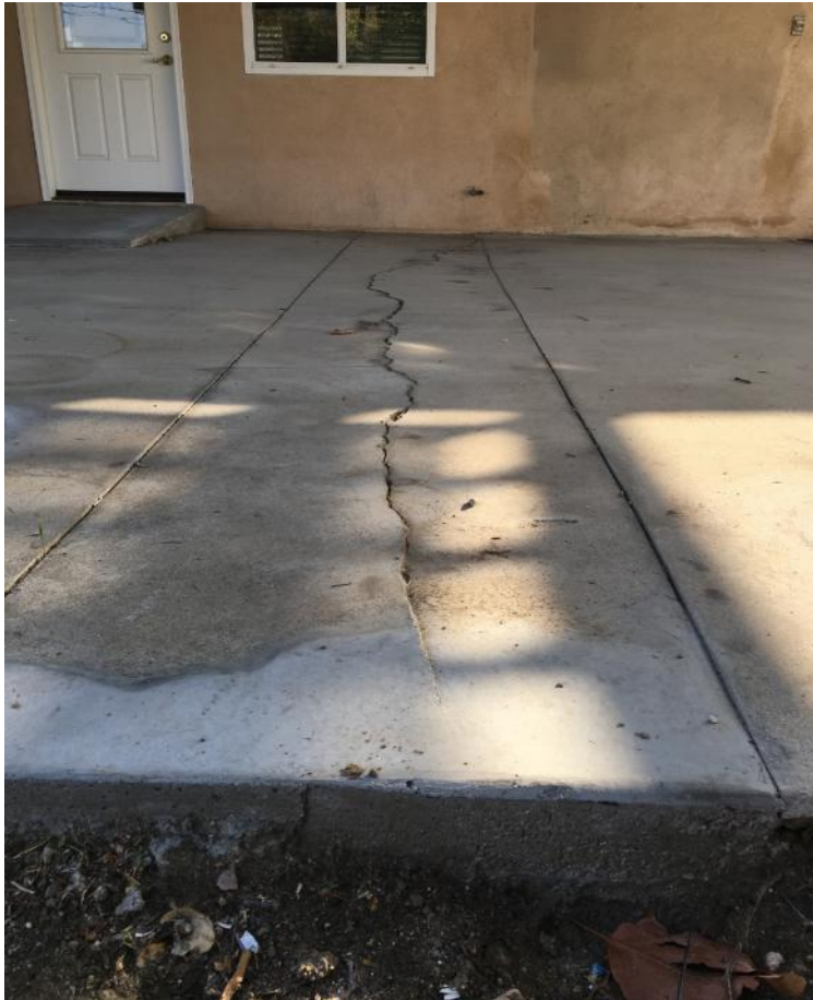
Photograph No. 10: Cracked patio slab on west side of residence at 1205 University Street
