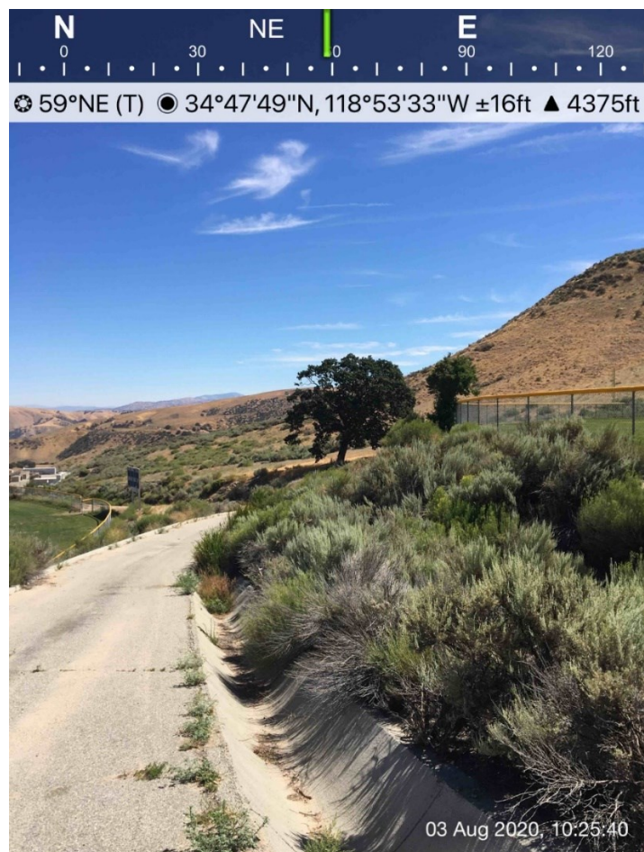
Photograph 76: FMHS v-ditch from tank site along existing road toward school.
