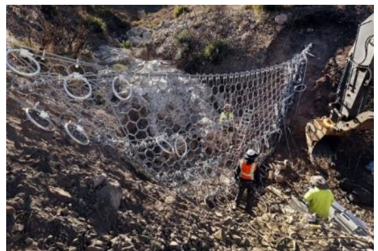
Photograph 3. Required maintenance activities would vary depending on the size and total volume of sediment or other debris captured by the debris nets. Minor debris accumulation maintenance would involve the use of hand tools (e.g., picks, shovels, and small hydraulic splitters). If major debris accumulation occurs, maintenance would require the use of heavy construction equipment.
