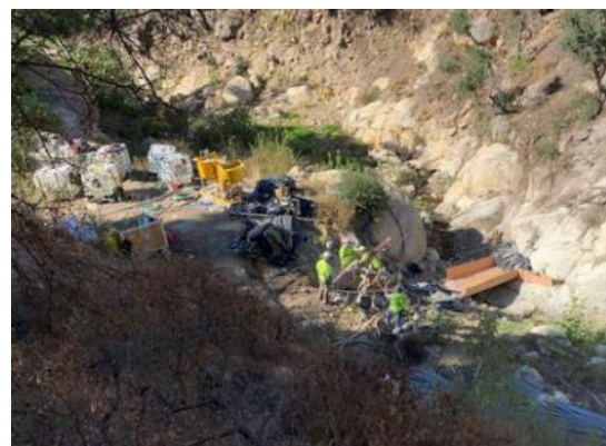
Photograph 7. During major maintenance activities, heavy construction equipment and materials would be airlifted to the debris net locations and staged in unvegetated disturbed areas, similar to the original installation activities (as pictured above at Buena Vista Creek).
