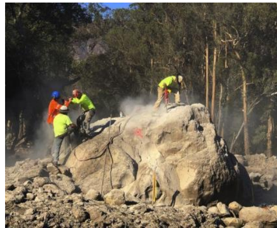
Photograph 8. Major maintenance events with major debris may require removal of large boulders using hydraulic splitters and excavators.
