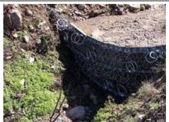
Photograph 5. In the event of major debris accumulation, heavy construction equipment would be required to remove the large boulders, rocks, tree trunks, branches, and other debris to restore capacity and function of the existing debris nets. (Photograph of captured debris within Camarillo Springs.)
