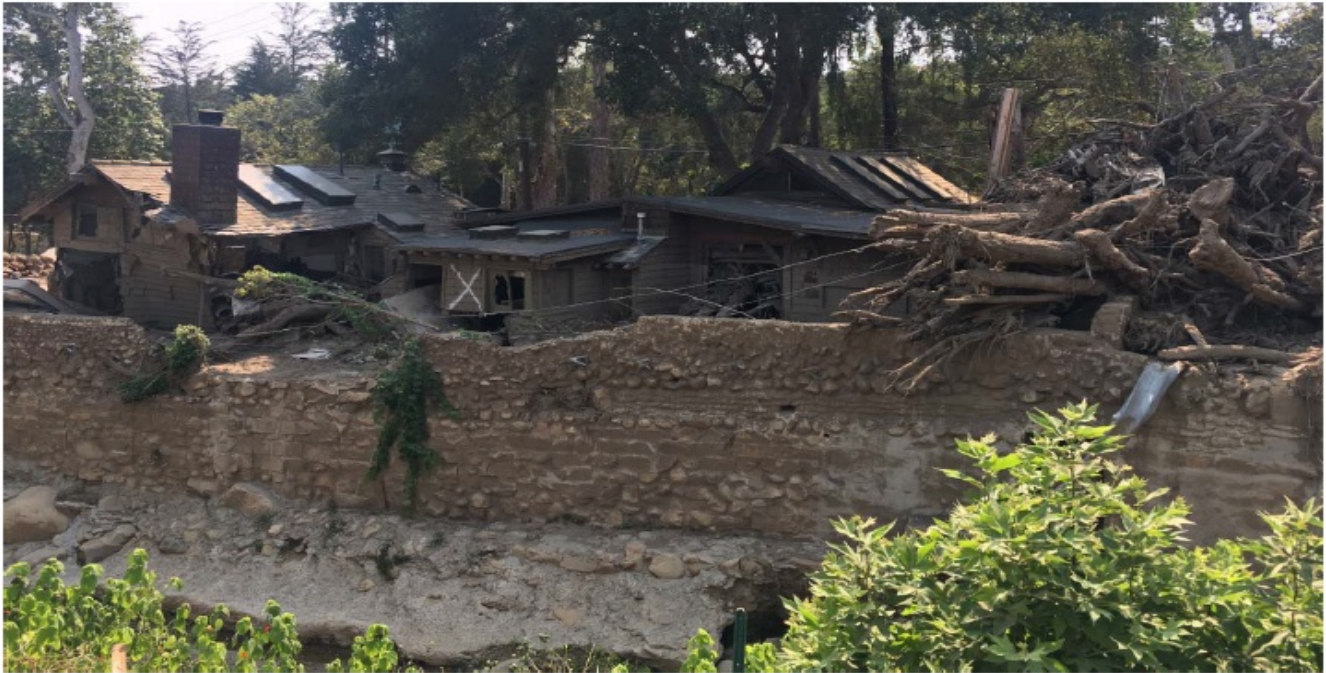
Figure 10. Woody debris immediately upstream of a destroyed home on Montecito Creek located approximately 2 km from the fan apex. BGC photo, July 2018, looking west.
