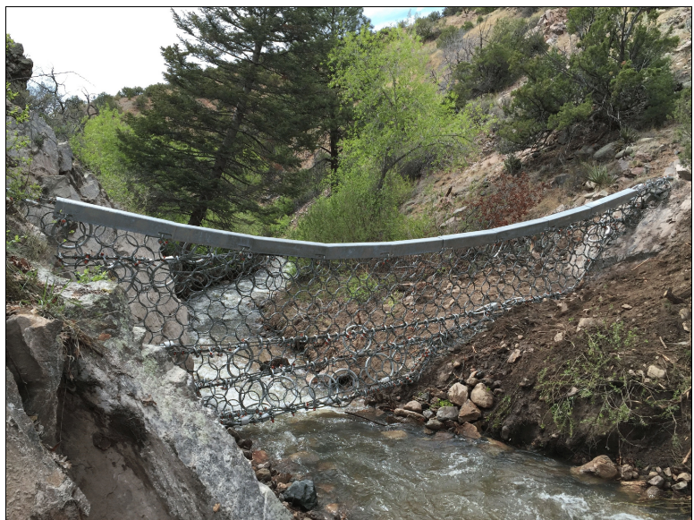
Figure 10. Post-fire VX net installed above running stream on the Nambé Pueblo, New Mexico. Note basal opening allowing water and fish passage beneath.
