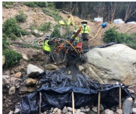
Photograph 18. During the initial installation of the debris nets, temporary secondary containment structures were successfully used to ensure that there were no accidental spills associated with heavy construction equipment. Similar BMPs would be installed during all maintenance activities involving the use of power tools or heavy construction equipment.
