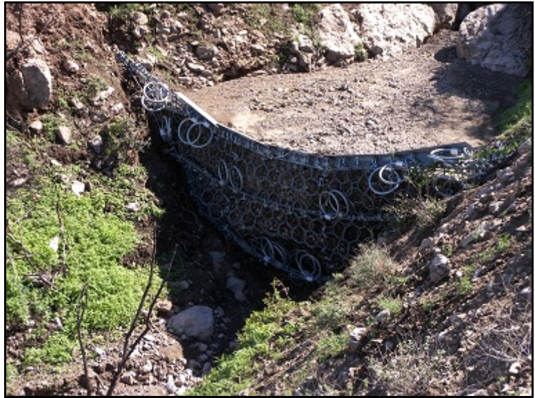
Figure 9. Geobrugg VX debris net protecting the community of Camarillo Springs, California. The net is easily cleaned after filling.
