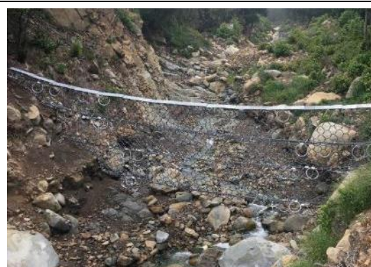
Photograph 2. Six Geobrugg flexible debris nets were installed within Cold Springs Canyon, San Ysidro Canyon, and Buena Vista Canyon. SY-18 (pictured above) was installed in San Ysidro Canyon in April 2019 under the original Emergency Permit issued by the County.
