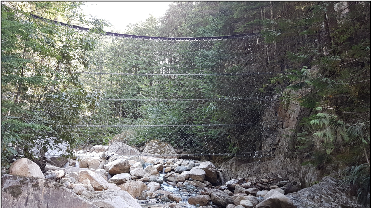
Figure 11. "Super VX" debris net installed in British Columbia, Canada. Note freeboard beneath net to allow stream flow and animal traffic. Basal opening freeboard is adjustable to eliminate construction excavation in stream channel.
