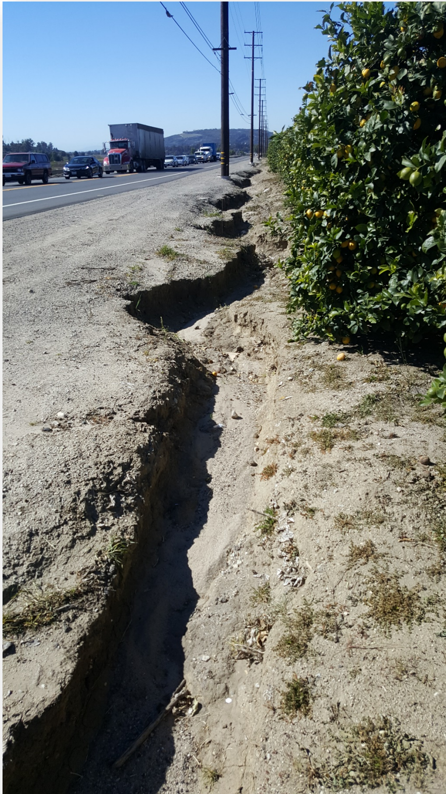
Figure 5: Shoulder Erosion
