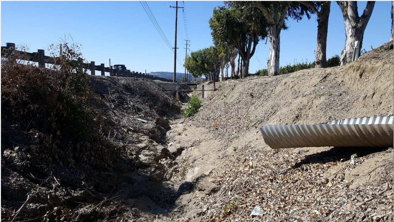
Figure 2: SR-118 Slope Erosion
