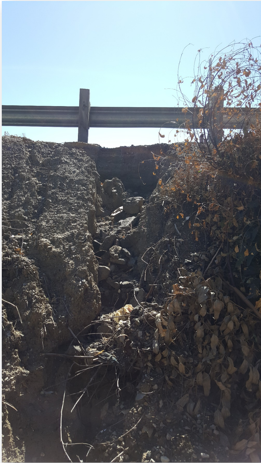
Figure 6: MBGR Damage
