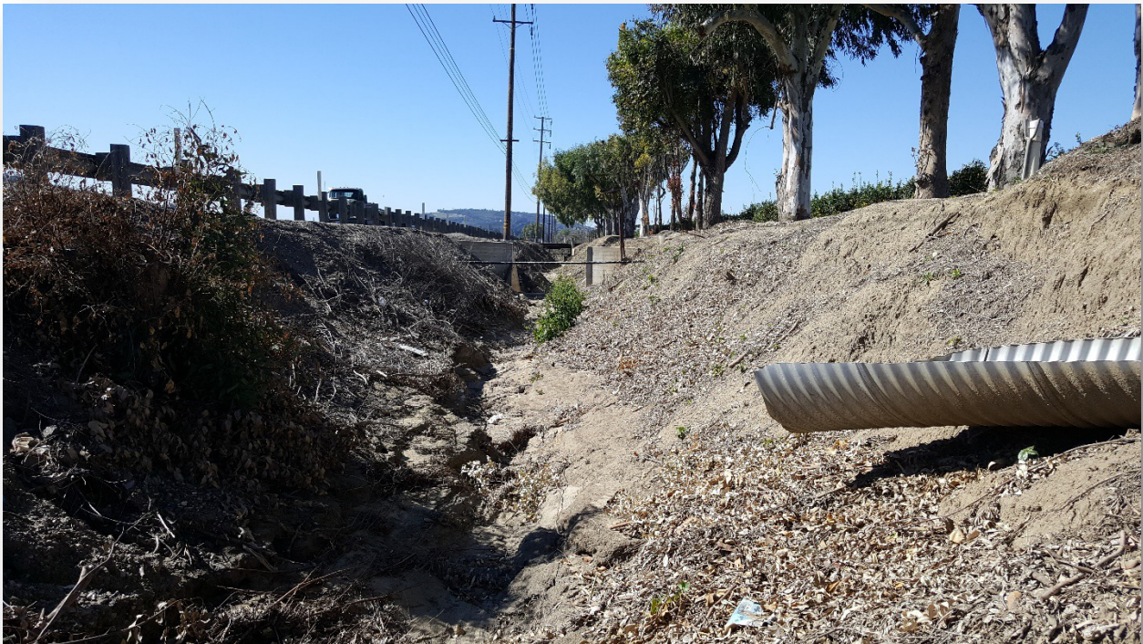
Figure 2: SR-118 Slope Erosion
