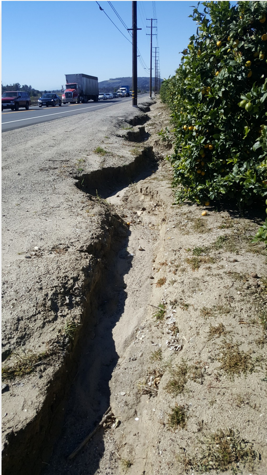
Figure 5: Shoulder Erosion
